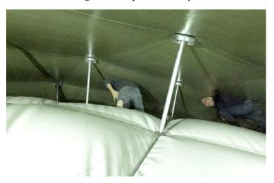
Fig. 2. Detail from a real-scale model. The cavity pins connect the Dome (lower layer) and the Tent (upper layer)
